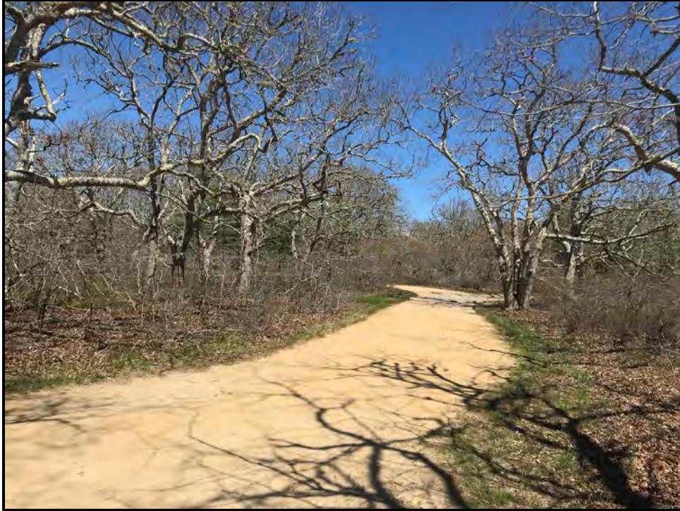
Figure 2.10. Example of an unsurfaced road.
